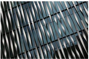
Low specific weight, aluminium plate and sheet can create structures with only 50% to 66% the weight of steel and only 15% the weight of reinforced concrete structures, all with the same bearing capacity. Aluminium lightweight structures require reduced shallower and simple foundations. Light weighting using aluminium has been extended into curtain walls, roofing and cladding, solar shading and even photovoltaic panels.
