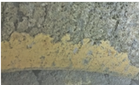
A PBond Solo 60 repair after 5 months in service
