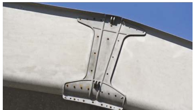
Detail of the cast aluminium junction between two mill-finished aluminium beam components formed from 4mm aluminium sheet. Note that the beams also serve as gutters to the roof panels.
